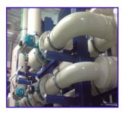
The PP-Pure<sup>®</sup> system uses a pigmented random copolymer polypropylene resin (PP) for its pipe, fittings and valves. PP-Pure<sup>®</sup> pipe and fittings are extruded and molded in a standard facility. The parts are immediately cleaned in an automated six phase hot UPW system.
